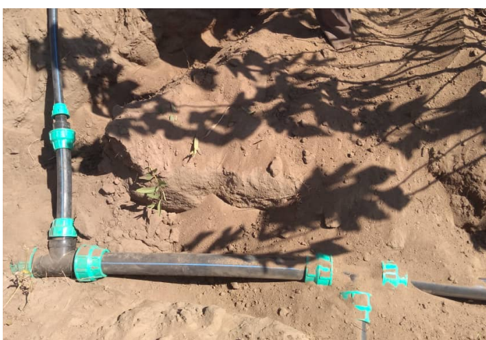
Installation of irrigation pipes
